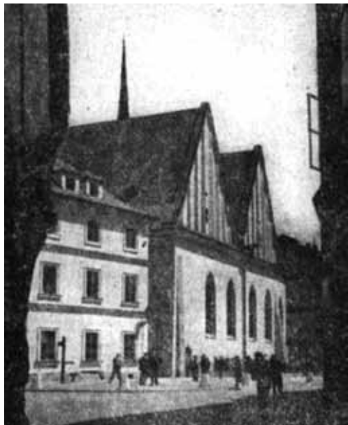
Bethlehem chapel in Prague after reconstruction. Condition in 1955. (1955). Večerní Praha , 1, 8, 9. 4., 1.
