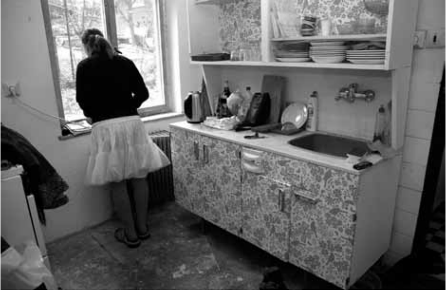
Kitchen prior to reconstruction – semi-detached house.
