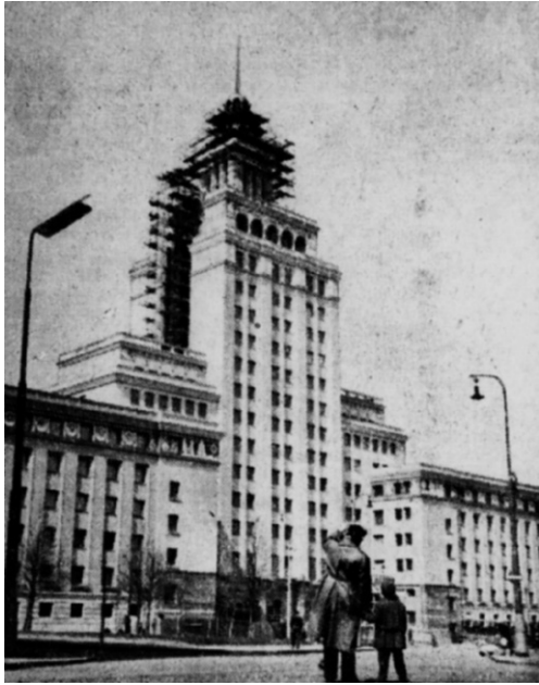
First high-rise building in Prague. Hotel Družba in Podbaba (later Hotel International, today Holiday Inn). Condition in 1955. (1955). Večerní Praha , I, 21, 26.4., 2. Photograph E. Einhorn.
