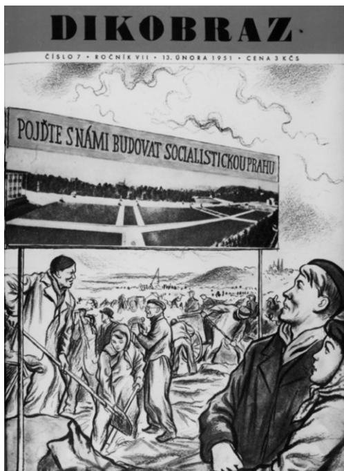
Construction site at Letná – the first important collective Prague building. Propaganda drawing O. Mrkvička. (1951). Dikobraz , VII, 7, 13.2., title page.
