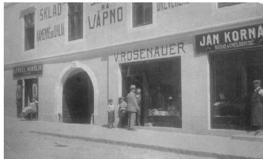
Picture No. 1: ORIGINAL BUILDING OF THE “U MIHÁLIKOV” BAKERY (BEFORE 1928)
